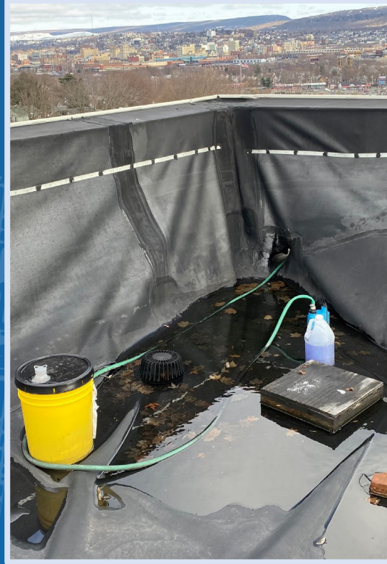
ROOF DRAIN & SUMP PUMP
