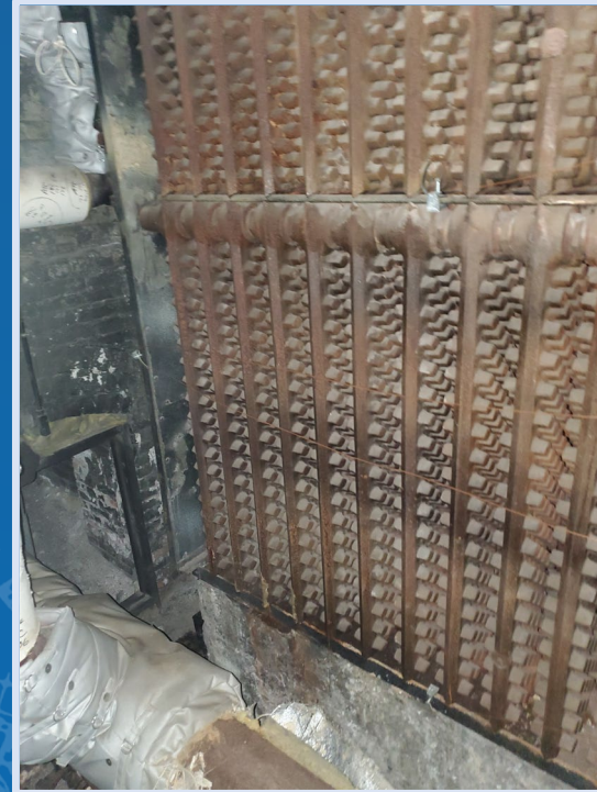
HEATING COIL FOR TEMPERING VENTILATION AIR
