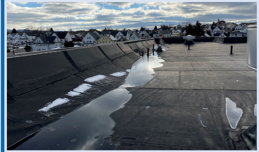
EPDM ROOFING SYSTEM
