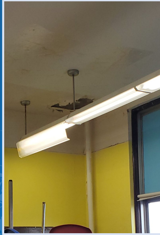
CEILING DAMAGE
