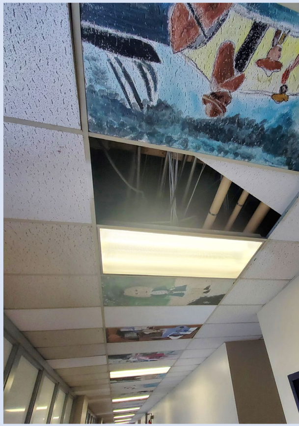
DAMAGED CEILING TILES
